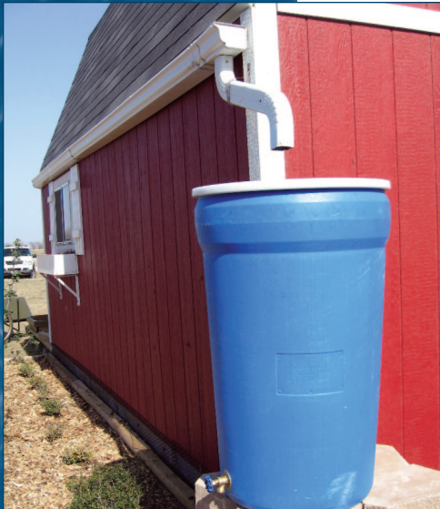
Figure 1. Example of rain barrel.
